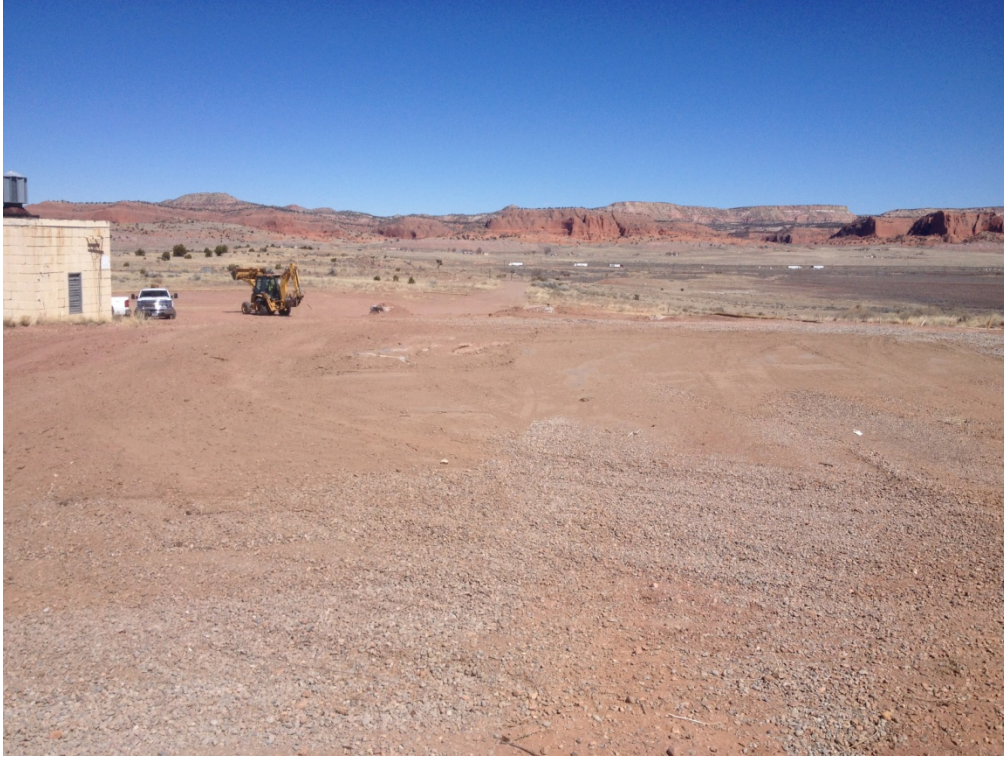
Photograph No. 11 March 09, 2016 – Backfill of excavated areas.
