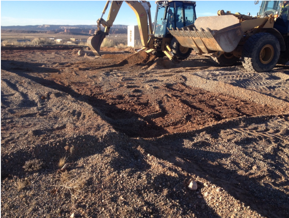
Photograph No. 9 December 02, 2015 – Secondary removal activities.
