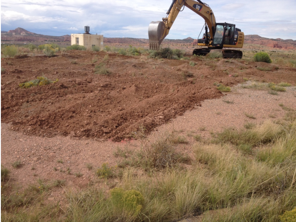
Photograph No. 3 September 01, 2015 – Soil stabilization process.
