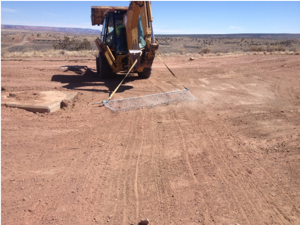
Photograph No. 12 March 09, 2016 – Preparing ground surface for seeding.
