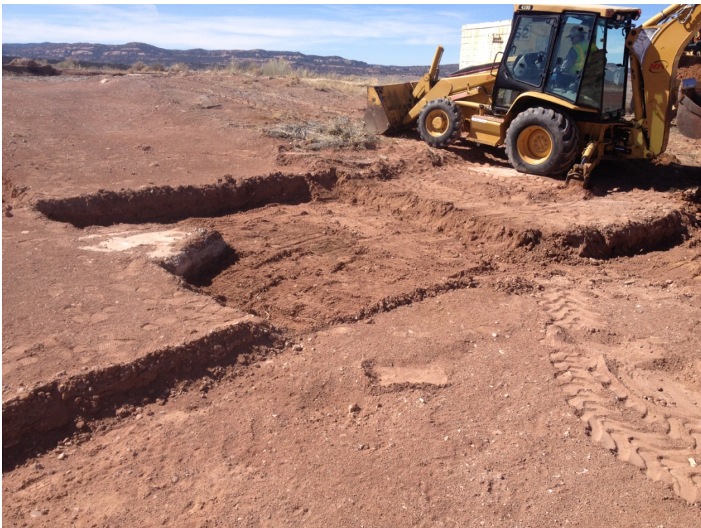
Photograph No. 10 February 24, 2016 – Final removal activities.
