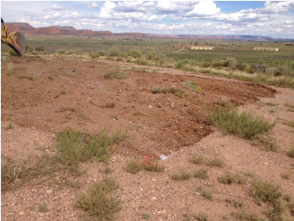
Photograph No. 4 September 01, 2015 – Soil stabilization process.
